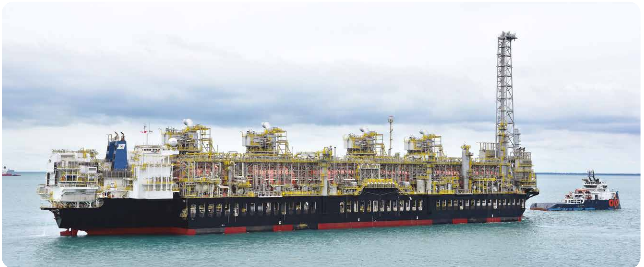
Sailaway of Gimi, the world's second converted FLNG for Golar LNG, following successful delivery of the first converted FLNG Hilli Episeyo in 2017
