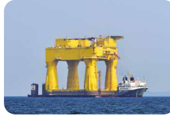
Sailaway of DoWin epsilon, a 900MW HVDC Offshore Converter Platform for TenneT
