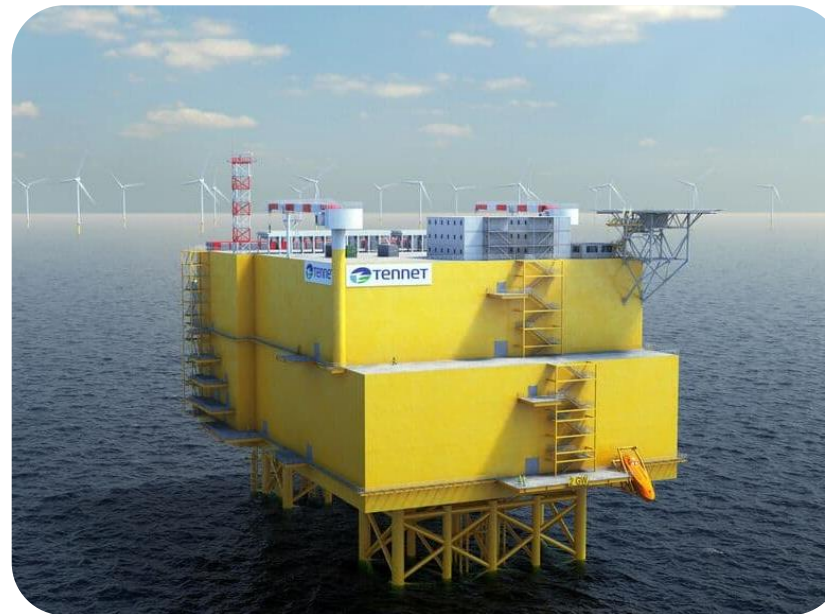
Illustration of TenneT 2GW HVDC substation
