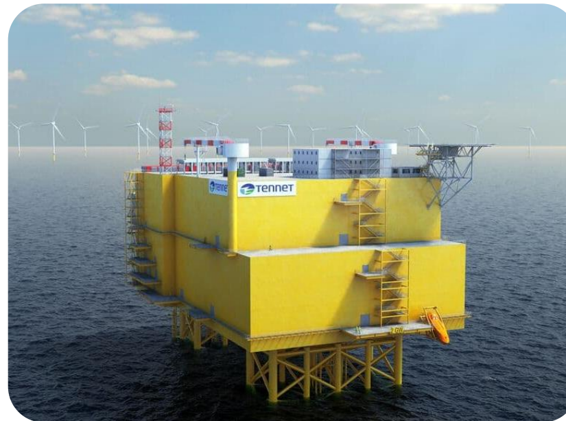
Illustration of TenneT 2GW HVDC substation
