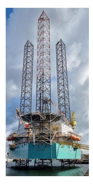
Captions: Built to world-class KFELS B Class design, the "AlSila" is capable of operating in water depths of over 400 feet with the ability to drill to depths of up to 30,000 feet for horizontal and vertical deep wells.
