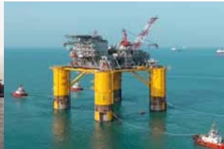
Vito , first floating production unit built by Sembcorp Marine
