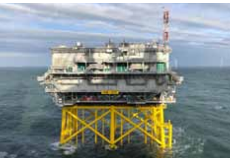
Hornsea Two Offshore Substation Platform for the world's largest offshore wind farm, Hornsea Two Offshore Wind Farm
