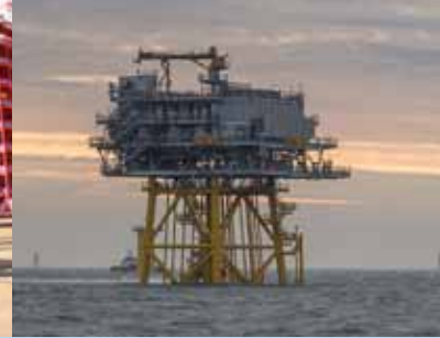
Dudgeon Offshore Substation Platform deployed for the Dudgeon Offshore Wind Farm
