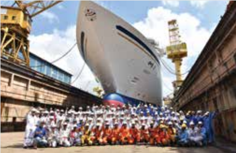
In March 2020, we completed the major upgrade of Asuka II, Japan's largest cruise ship, for NYK Cruise. The upgrade involved extensive refurbishment and scrubber installation.
