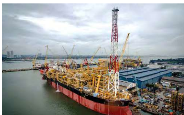
One of two FPSO conversion projects for the Kaombo field offshore Angola
