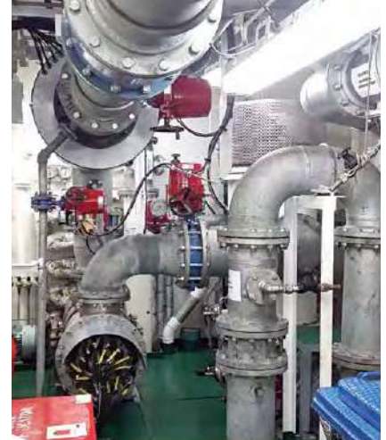
Another milestone achieved with the Ballast Water Management System development: Successfully completed US Coast Guard shipboard tests
