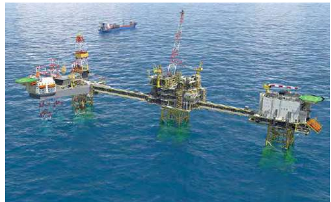
Sembcorp Marine's support of the high-pressure, high-temperature gas and condensate development in the Culzean field includes the engineering, procurement and construction of three fixed platform topsides, and construction of a floating storage and offloading vessel as well as a jack-up rig
